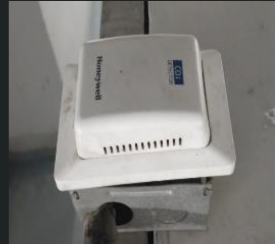
Duct mounted return air CO2 sensor for IAQ application
